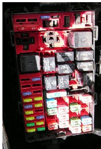
This is a typical arrangement for the fuses inside the fuse box
